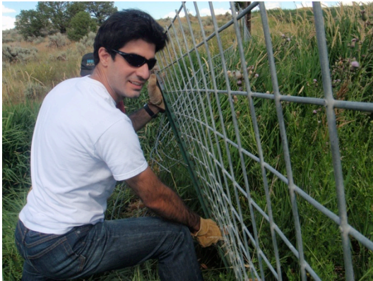
Graduate student intern Raffi Andonian repairing a protective fence around the Yellow Jacket site in southwestern Colorado for The Archaeological Conservancy, July 2011.
